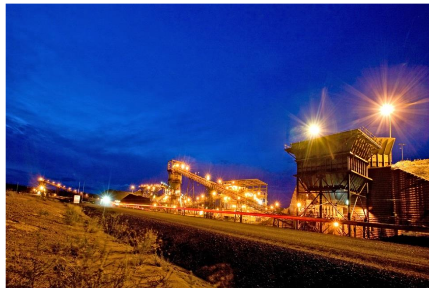
The coal handling and preparation plant in Coppabella Mine
